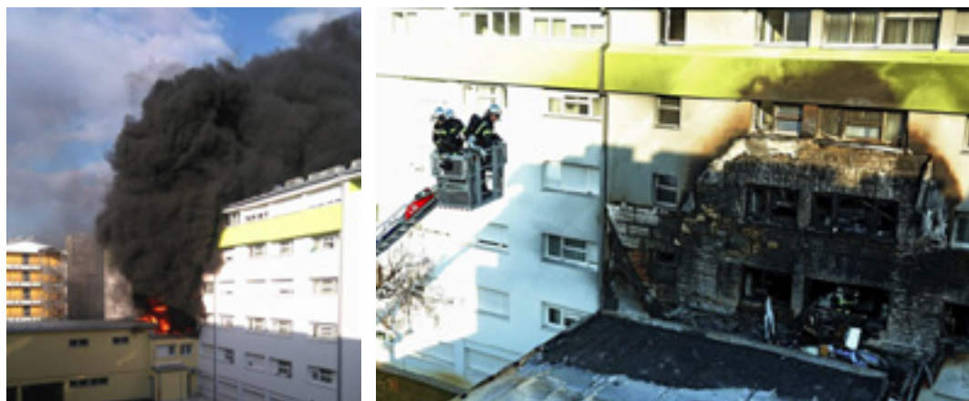
Figure 16. a) Fire in student dormitory b) the façade after the fire was extinguished [11], [25]
