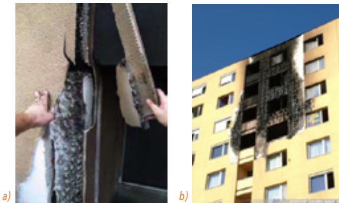
Figure 13. Consequences of fire on the façade of the residential building in Miskolc, Hungary
