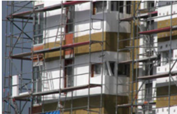
Figure 31. Example of a vertical fire barrier on a façade
